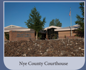
Nye County Courthouse
