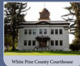
White Pine County Courthouse
