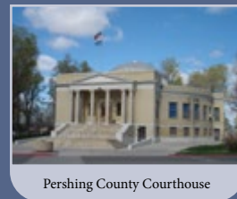
Pershing County Courthouse
