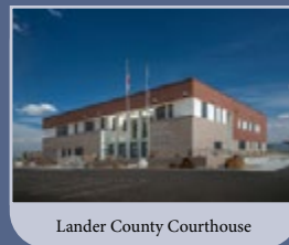
Lander County Courthouse
