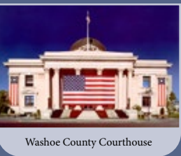
Washoe County Courthouse
