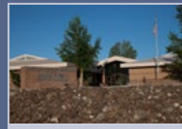
Nye County Courthouse
